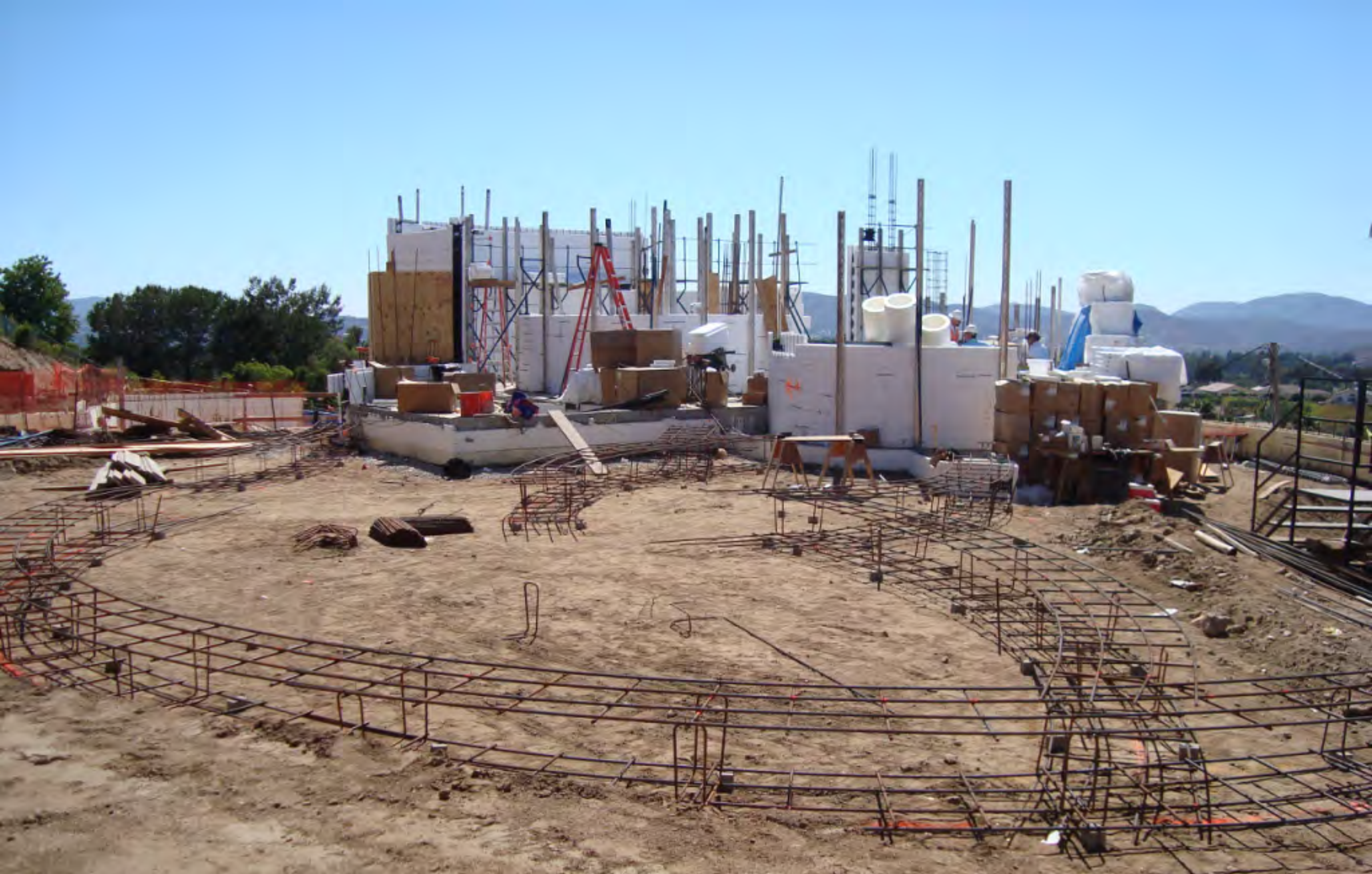
Rebar cradles prior to IntegraFooting installation.
